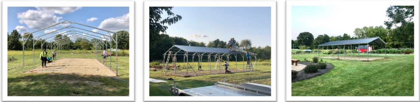
Figure 2 - Assembly process and finished shelter
